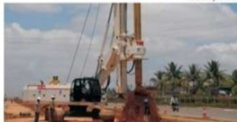
Hydraulic Piling Rig
