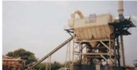
Hot Mix Plant
