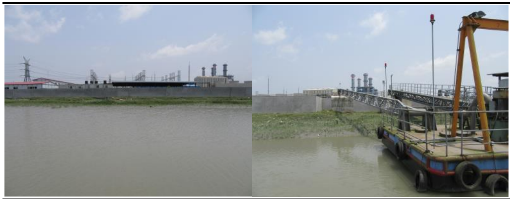
Figure 0.11 Existing Bhola I Premises
