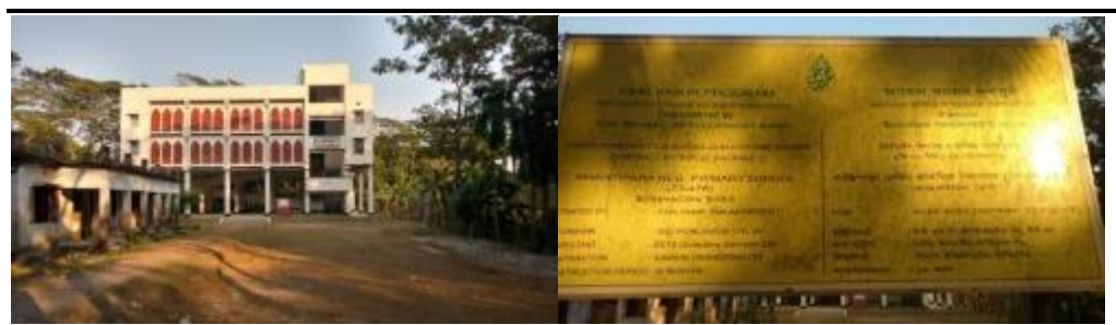
Figure 5.17 Cyclone shelter in Shantipara Village, Kachia
